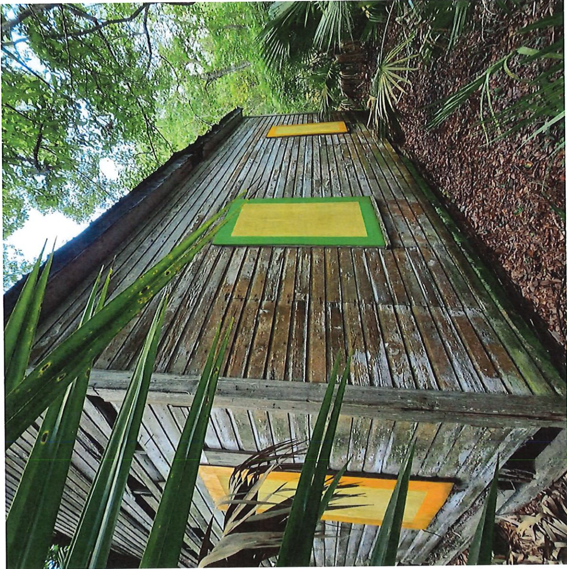
Today: Original Dwelling Right side Facing into Interior of Lot 10
