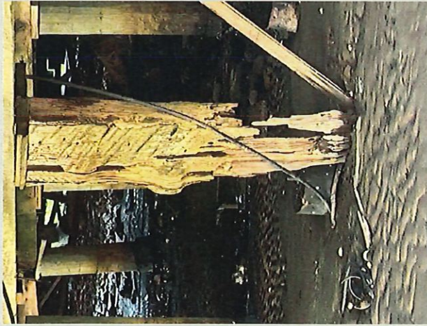
Deteriorated Piling
